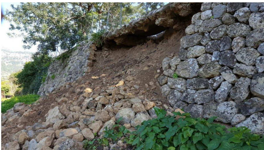
Figure 9 - Collapsed dry-stone wall as a result of a lack of maintenance. Source: Author's research.
