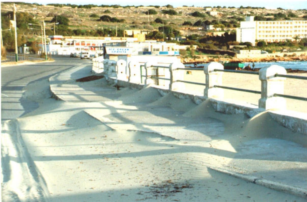
**Figure 4: Aeolian transport of beach sediment and sea-weed fragments (foreground) beyond an artificial sea-wall (centre - right of the picture) on to the coast-road bordering the back-shore of the beach at Ghadira Bay, north-western coast of Malta.**
